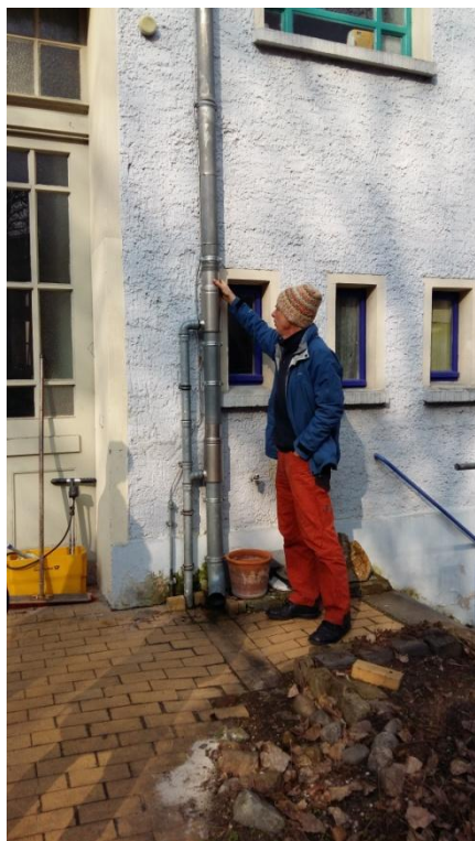
Pic. 9 RW collecting pipes with incorporated filter; Author: Laura Palau
