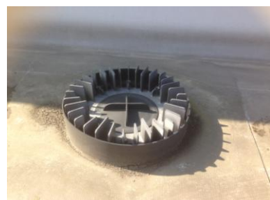
Pic. 13 Roof rainwater collection overflow inlet; Author: Lina Suleiman
