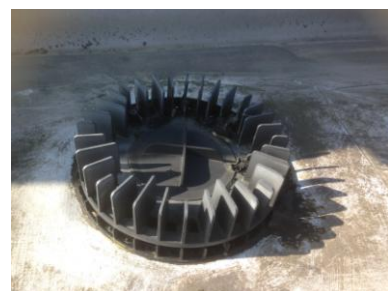
Pic. 14 Roof rainwater collection inlet; Author: Lina Suleiman
